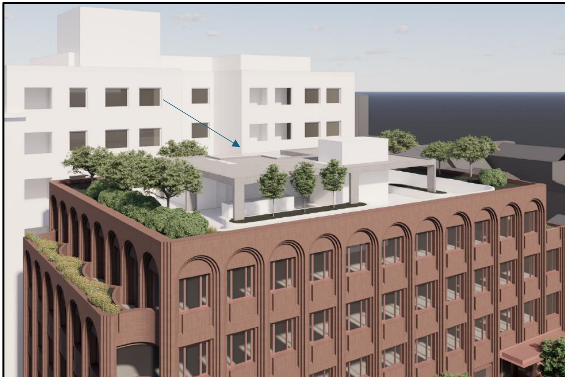
Figure 9: Excerpt from the architect's design report, which shows the recessed nature of the uppermost 6th storey and associated pergola, lift and fire stair components, which are primarily responsible for the height variations. The perimeter planting will also assist in minimising the visual impact of the upper-level components when viewed from public vantage points around the site.
